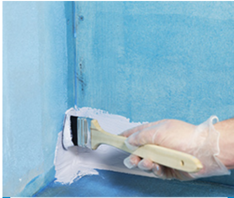
Installation of Mapei IC/EC corner gasket by using Mapegum WPS
