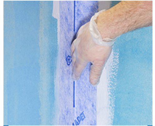
Installing Mapei ST sealing tape by using Mapegum WPS, wall
