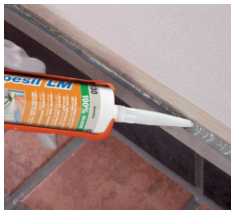
Sealing of exterior stone cladding
