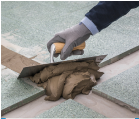
Filling a cable run with Planipatch Xtra Zero
