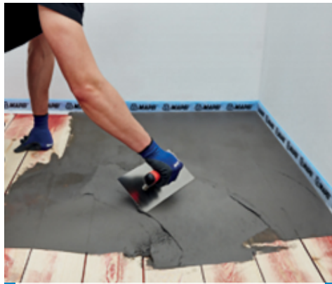
Application of Planipatch Xtra Zero + Latex Plus on wooden substrate
